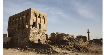
Ruins of abandoned houses at Al Jazirat Al Hamra Photo credit: Stevenmcombe/CC 4.0
