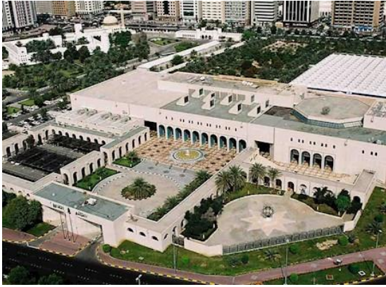
The renovated Abu Dhabi Cultural Foundation Centre. Photo courtesy: Abu Dhabi Culture
